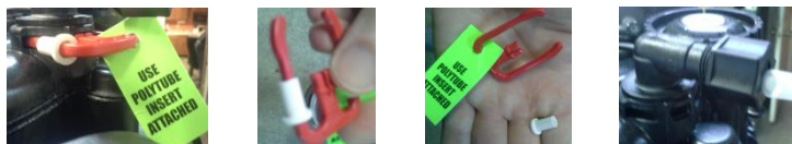
Figure 14: Installing Brine Line Polytube
