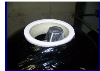
Figure 8: How to Block Distributer Tube
