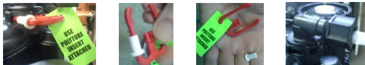
Figure 13: Installing Brine Line Polytube
