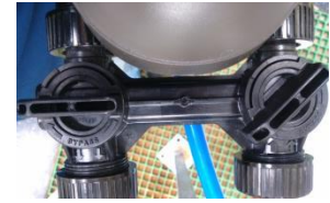
Figure 14: Opening bypass valve's inlet
