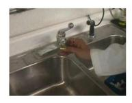
Remove the aerator from the end of the faucet; make sure all rubber seals are also removed.
