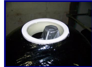
Figure 7: How to Block Distributer Tube
